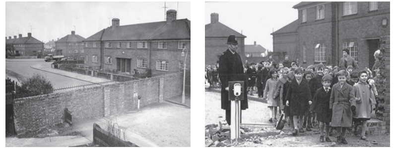
One of the Cutteslowe Walls: (left) standing, and (right) demolished.
